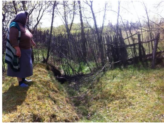
Figure 5. Surface affected by the underground mining
