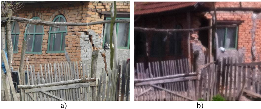
Figure 4. Buildings affected by the underground mining a) 07.1.2016 b) 26.10.2016
